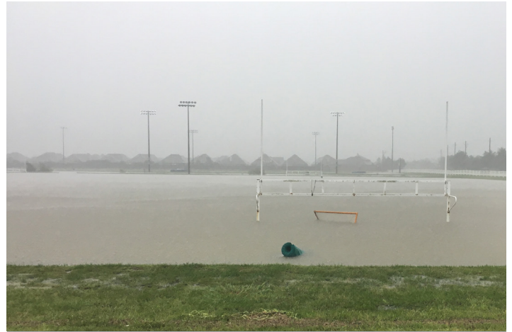
FIGURE 30. AN ATHLETIC FIELD AT A FRIENDSWOOD, TEXAS JUNIOR HIGH SCHOOL BEING USED AS A DETENTION POND DURING HURRICANE HARVEY, 2017. SOURCE: W. HIGHFIELD, TEXAS A&M.
