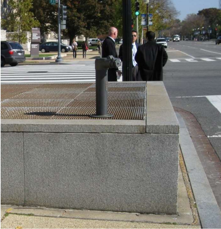
FIGURE 32. PERMANENT PROTECTION FOR WASHINGTON METRO SUBWAY VENT. SOURCE: WASHINGTON METROPOLITAN AREA TRANSIT AUTHORITY.
