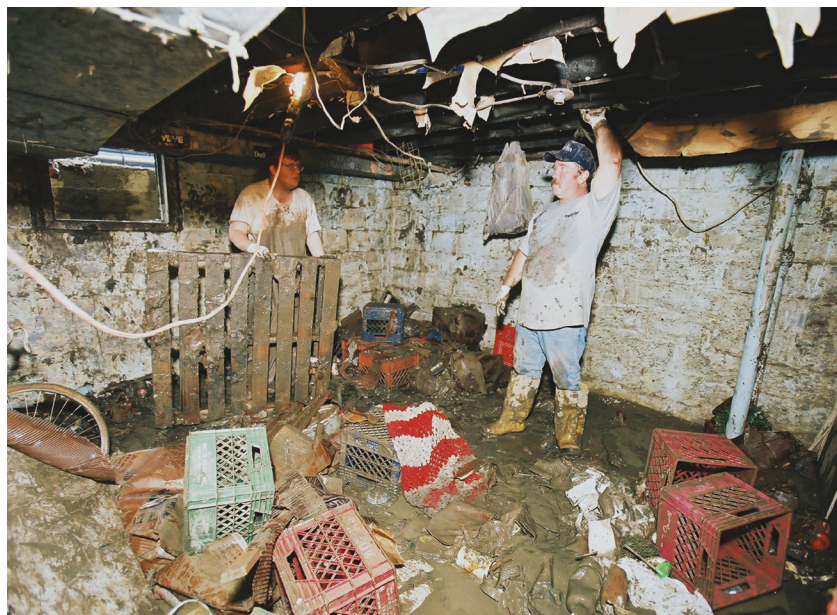
FIGURE 7. BRIDGEVILLE, PENNSYLVANIA RESIDENTS MUCK OUT THEIR BASEMENT AFTER A FLASH FLOOD. SOURCE: FEMA NEWS/PHOTO BOB MCMILLIAN.
